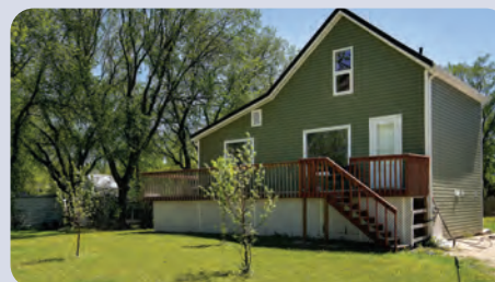
220 Kennedy W - MORRIS 945 sq ft, 3 bedroom double lot, upgraded foundation
