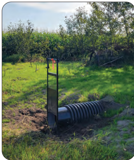
In the Morris Norquay Sub-District, Alan Richardson installed a gated culvert with help from the RBWD to regulate wetland water levels.
